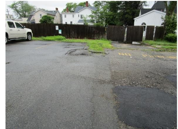
Pervious pavement can be installed to decrease the pooling and erosion caused by the pitch of the pavement and the downspouts leading to the northeast corner of the parking lot. Downspout planter boxes can also be installed to capture runoff from the rooftop. A preliminary soil assessment suggests that the soils have suitable drainage characteristics for green infrastructure.
